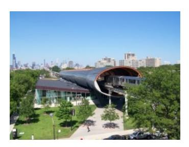
Chicago has the third busiest and second longest rail mass transit system in the country. It is known as the "L" for "elevated" because most of the system is on an elevated structure. The train station at the Illinois Institute of technology uses curved steel beams to form a tube which muffles the noise of the "L" as it
