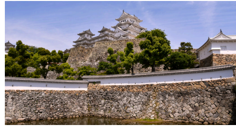
fig 1. Himeji Castle, constructed 1608. Himeji, Hyōgo Prefecture. Photo by Dr Mark Erdmann.[/caption]
